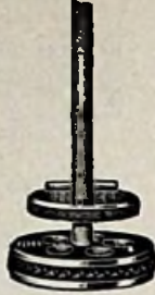
Fig. 151 Flax Packed Plunger
